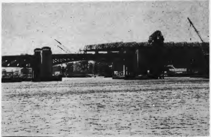
TIGHT SQUEEZE - The Fore River Bridge Replacement Action Team [BRAT] favors the building of a new Fore River Bridge in order to maintain the Quincy shipyard's competitive market position in future years. The present bridge has a horizontal opening span of 175 feet, sufficient to permit safe passage of ships with a beam of less than 150 feet.
